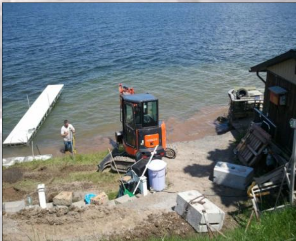
Shoreline construction adjacent to West Lake Road during the summer of 2014. The contractor failed to utilize sediment control which resulted in a plume of sediments into the Lake.
