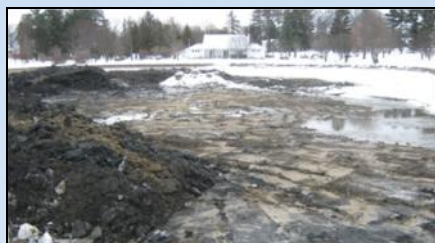
Floor of the pond with the material windrow ready for removal.
