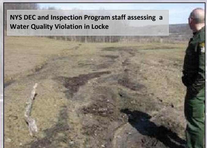
This steep slope was not vegetated after clearing in late 2013, resulting in severe erosion during the spring of 2014, transporting tons of soil offsite, directly to Owasco Inlet. Acting with urgency, the landowner, SWCD, and Inspection Program staff took measurable, timely steps towards stabilizing the site and eliminating the damaging sedimentation created by the erosion.
