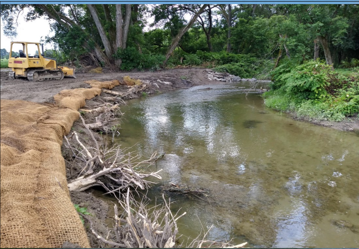
During construction, toe-wood protection with biomass plantings.
