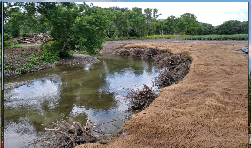
During construction, toe-wood protection with biomass plantings.
