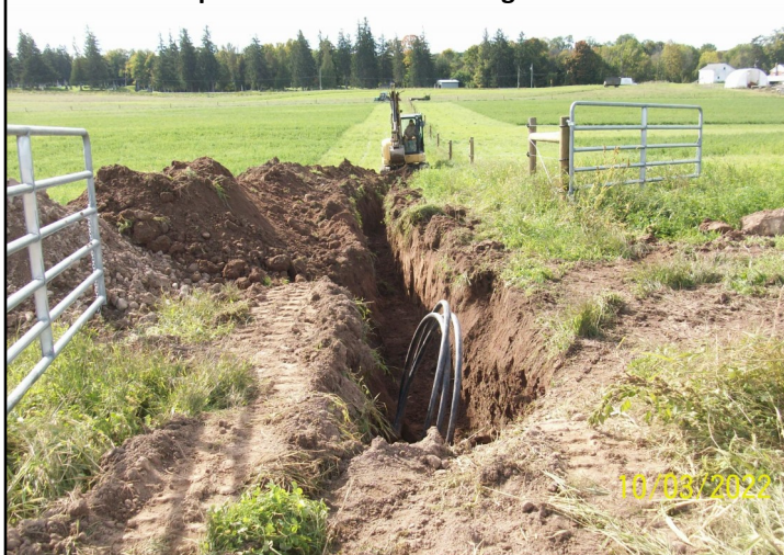
Example Waterline and Fencing Installation
