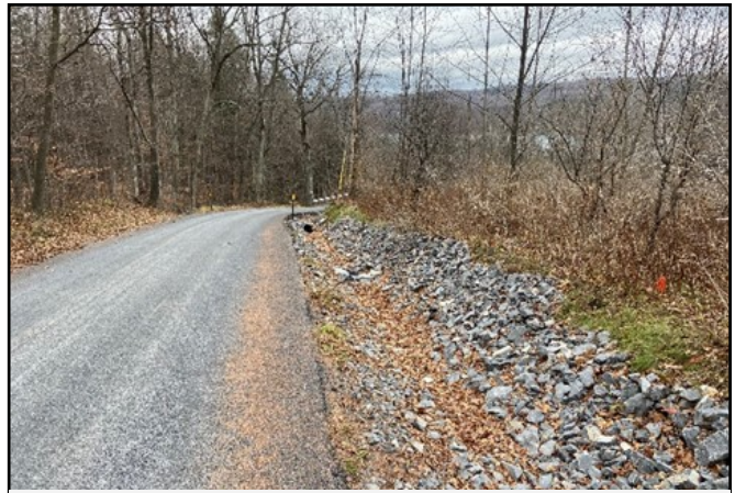
After picture showing the final stabilized ditch
