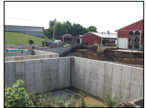
Above/Below: Construction of the storage, showing attachment to the existing storage.
