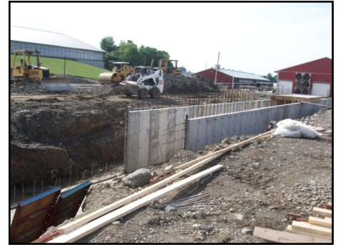
Above/Below: Construction of the storage, showing attachment to the existing storage.
