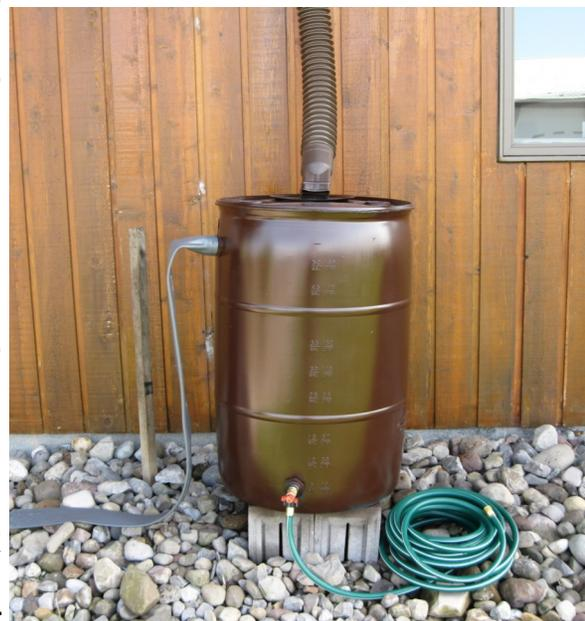
downspouts for winter, so we unscrewed what was there and replaced it with a flexible downspout we purchased from the local home store. There are also commercially made diversion spouts that can be fitted into your gutter system. These switch flow from barrel to spout with a flick of a lever. One even uses back-pressure to sense when the barrel is full and then sends the run-off down the down spout.
