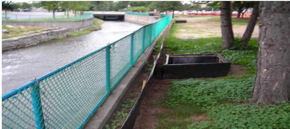
Above: One form of erosion and sediment control practices used on Market Street in Auburn, NY.
