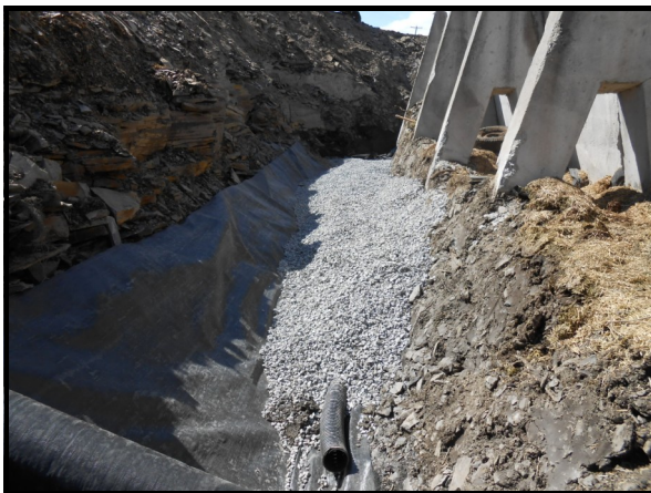
Above : Low flow collection system surrounding the bunk silo.
