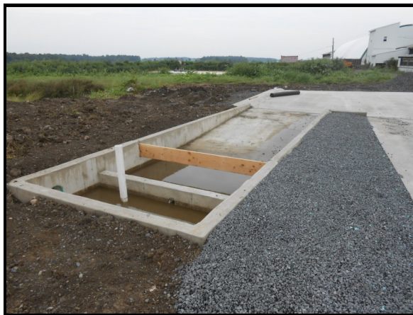
Above: Concrete high flow/low flow separator.
