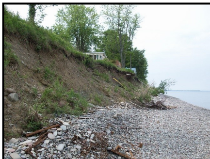
Before Project Commenced
