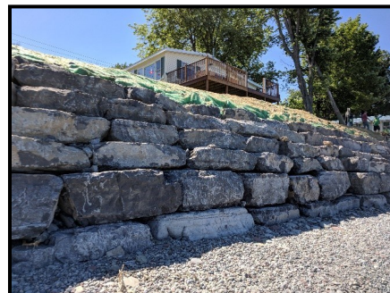
After Project Completed
